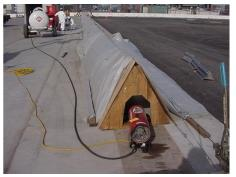
Hot Weather Grouting: [High temperatures accelerate set, decrease working time, and accelerate strength gain of epoxy products. The procedures below may compensate for these conditions.]
